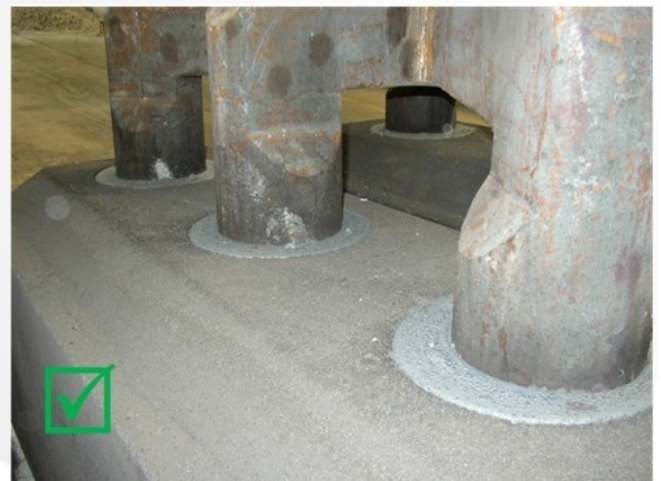
Figure 4: Correct cast iron application.
